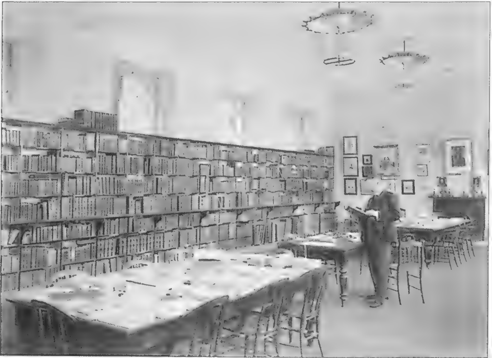
Fig. 11. The Royal Society of Tasmania Library and Members Room (formerly the Tasmanian Room), 1902. J.W. BEATTIE, PHOTOGRAPHER. TMAG: Q1989.49.1
